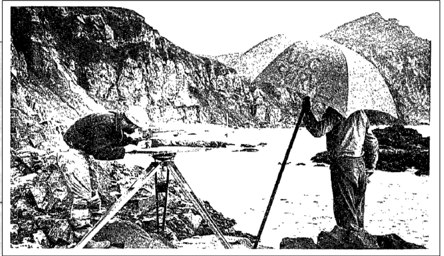
surveying with a planetable (Shalowitz 1964)
