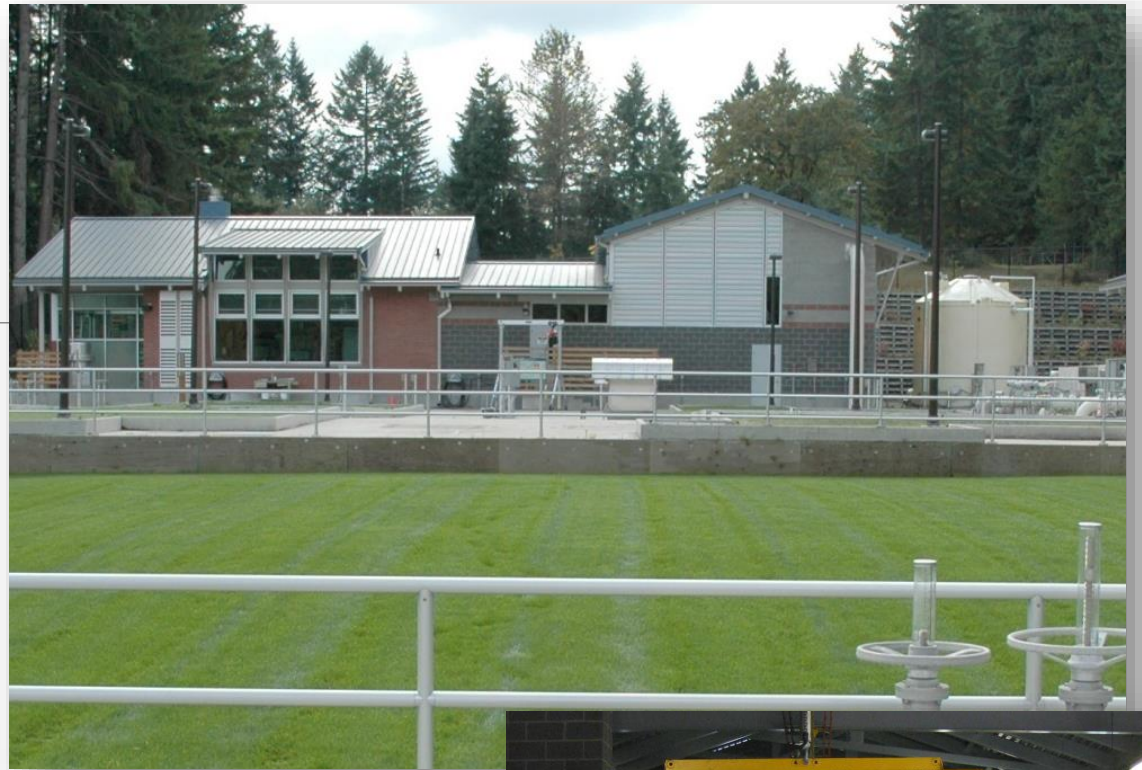
Martin Way Reclaimed Water Plant
